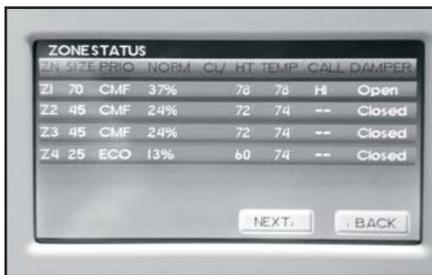
From the 'Zone' screen, press next. This screen shows the information the IntelliZone2 • 24V system is sending to the heat pump.
